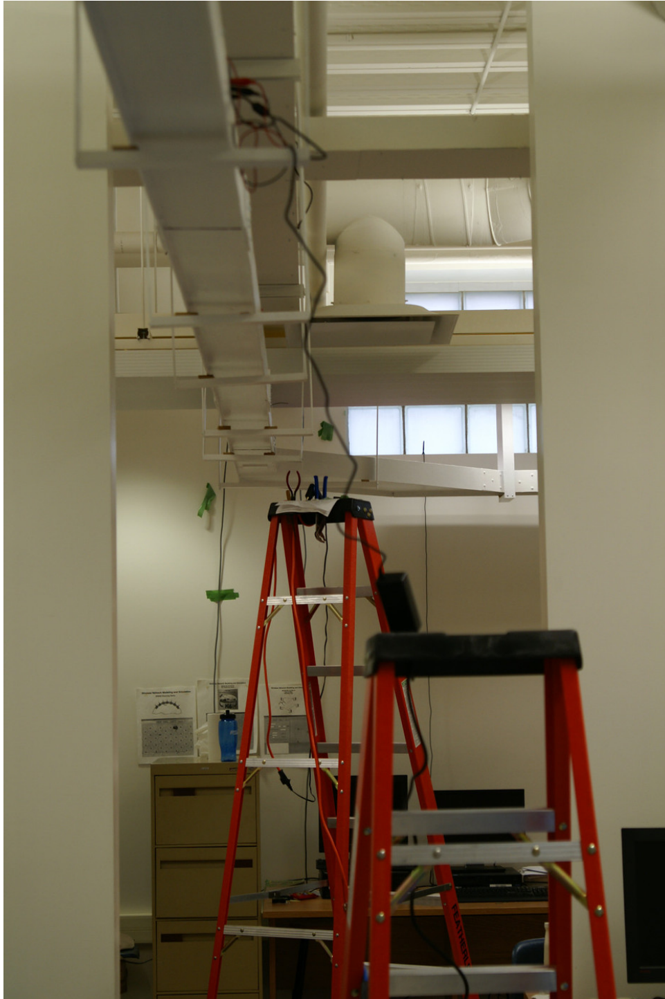
Figure 5.3: General view of train track in ITB214.
